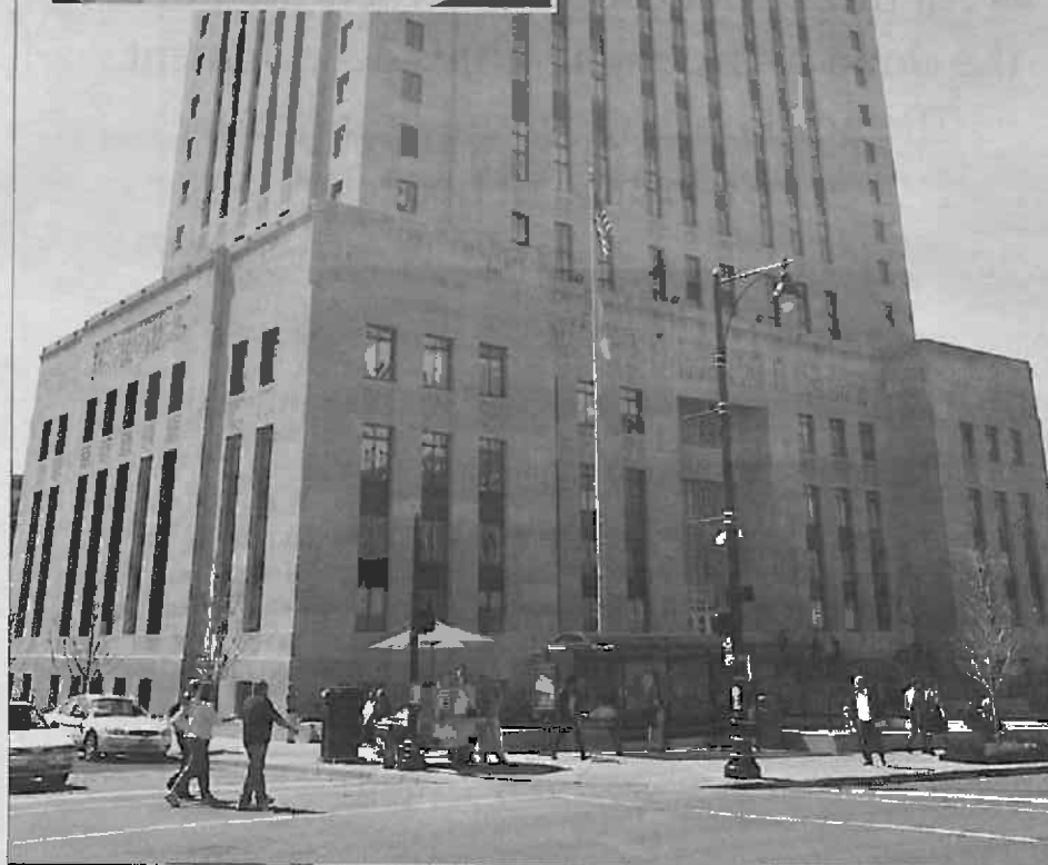
The Jackson County Courthouse was the site of a trial over whether workers were harmed by asbestos at the Jackson County Courthouse. Above, a notice informs the public that the air in the courthouse has cleared state and federal standards. Photos by Scott Lauck
